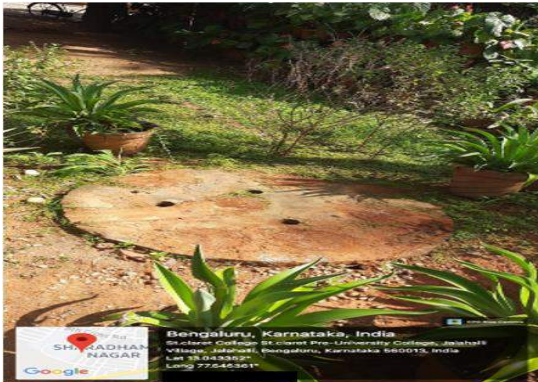
Figure 15: Storage Tank for Rainwater
