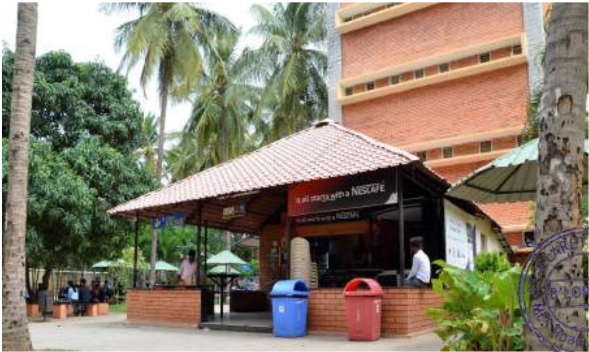
Figure 3: Canteen on premises
